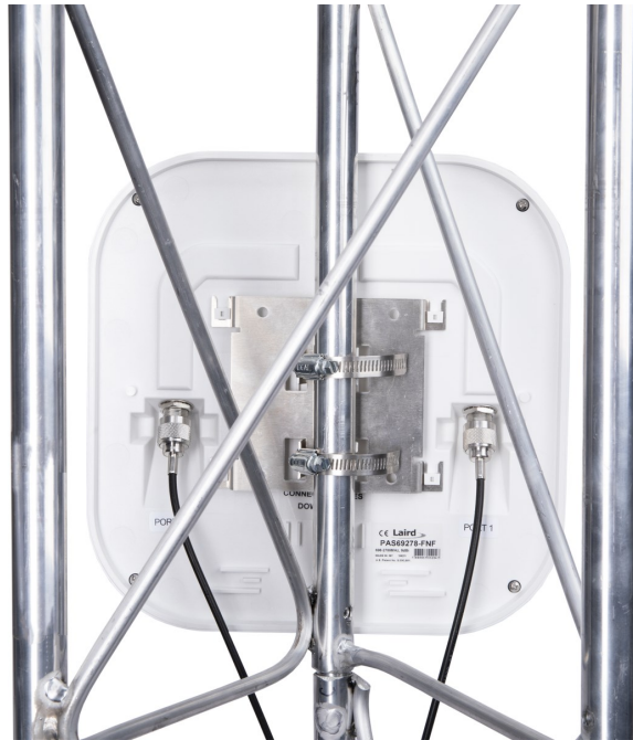
FIGURE 5-2. 38485 mounted on a tower
